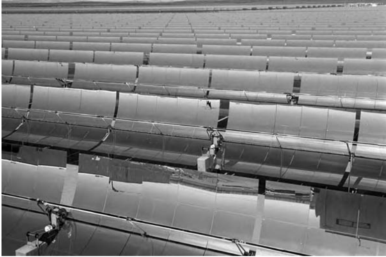
FIGURE 2.5 Solar collector field at a SEGS plant located at Kramer Junction, CA. (Photograph courtesy of Sandia National Laboratories.)
