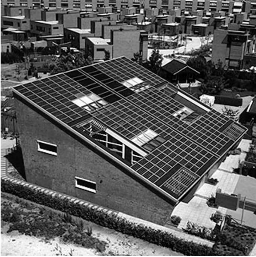
FIGURE 2.3 Roof-mounted Dutch PV subdivision, Nieuwland, in Amersfoort.
